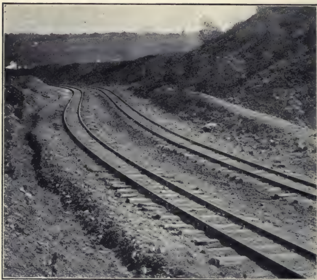
FIG. 12.—Well-laid narrow-gauge reverse curve.
